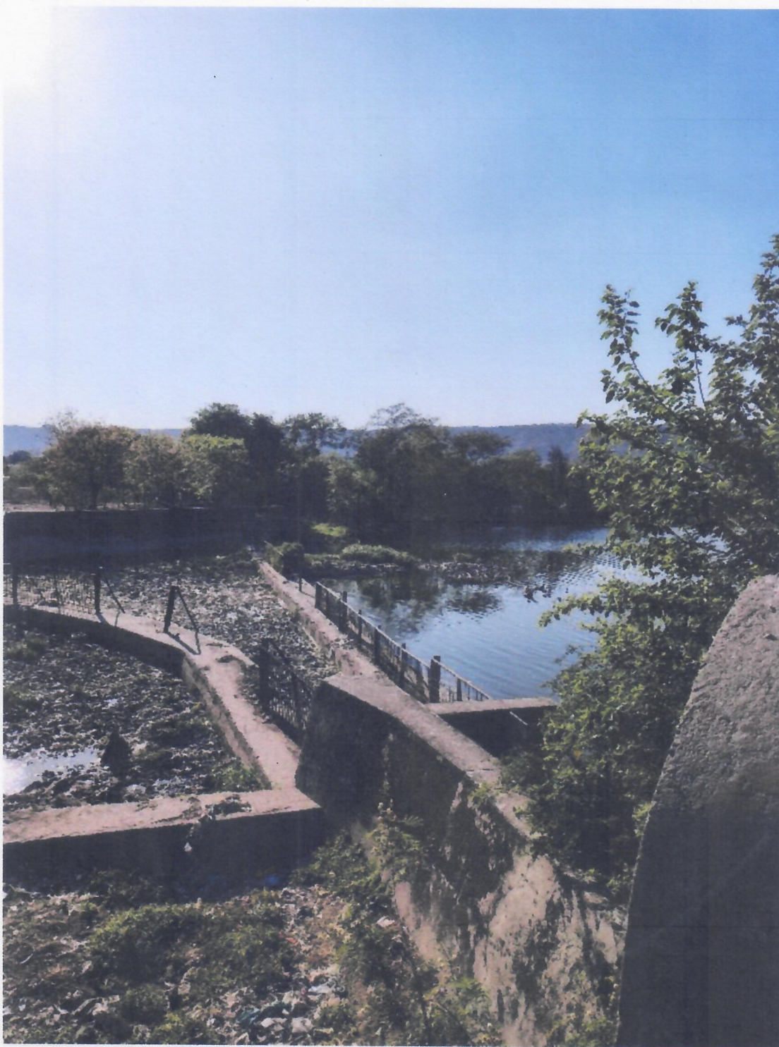
Figure 3: View of the Jal Mahal Lake and Nagtalai Nala from the entry towards Alwar Jaipur road
